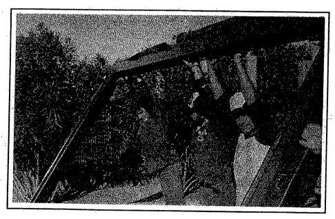
If the fork lift is available, power posts may be set upright and POWER BEAM lifted and set in place.
