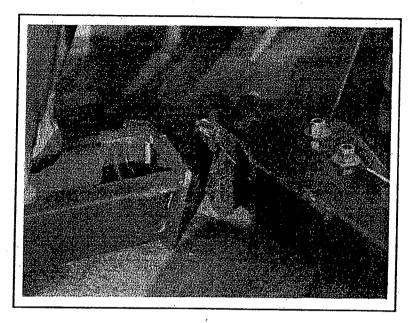
Tighten all bolts and drop chains through slots in top of power posts. Lift POWER BEAM assembly to an upright position placing mounting pads into corners of the chalk line layout.
